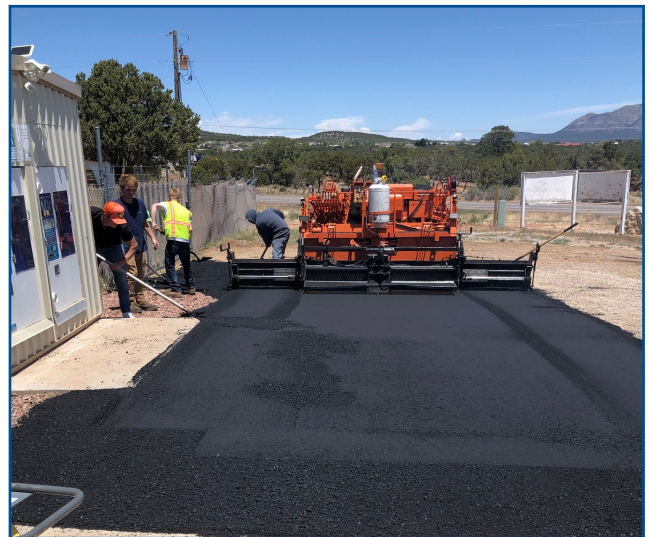
Asphalt crews pave the parking lot in May
