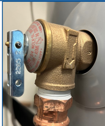
If blue lever pops, it could be a sign of high water pressure
